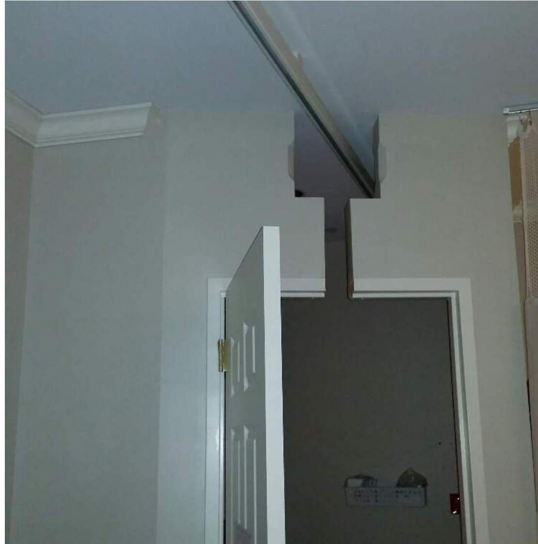
Safe resident/patient handling track installed to ceiling.
